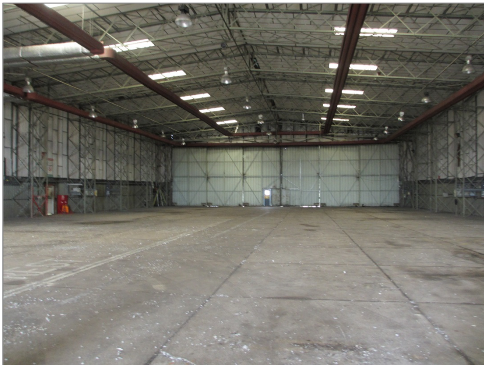
Figure 18: First cargo hangar interior
