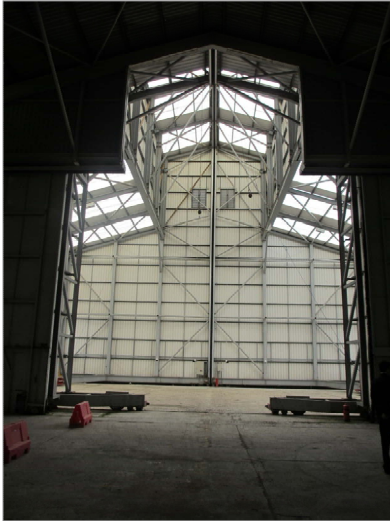
Figure 16: Bespoke tail enclosure of hangar
